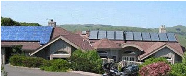
House with solar energy panels
